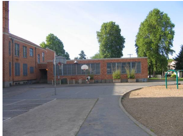
South elevation addition
