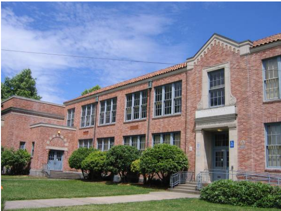
West elevation facing southeast
